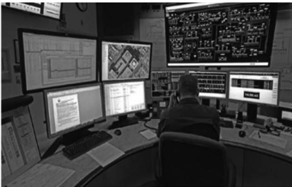
Figure 05: Distribution automation, a new effort
